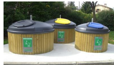
Figure 68: Exemple de conteneurs poubelle semi-enterrés (Source: Google Image)
